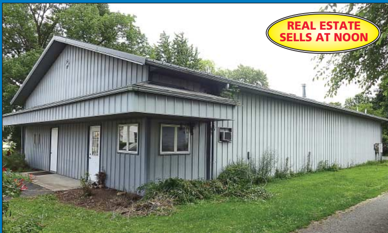
3,486 Sq. Ft. Morton Buildings Light Industrial Building on Approx. 0.80 Acres
